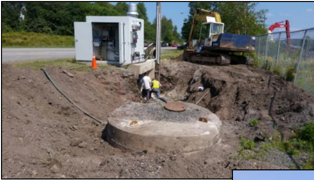
Contractors realigning pipes, replacing sensors and installing new pumps at the Ball field lift station. Work was also completed at the Market Street lighthouse and Sinclair station.
