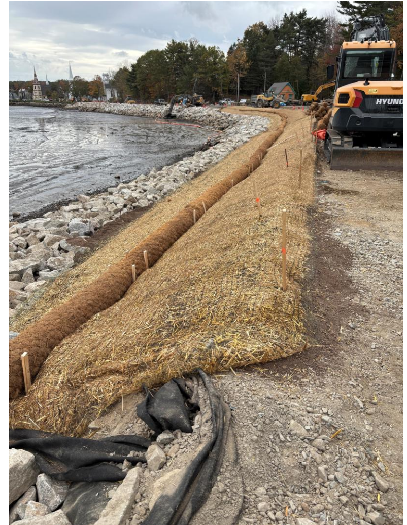
Construction of vegetated bank with rock toe at Mahone Bay
